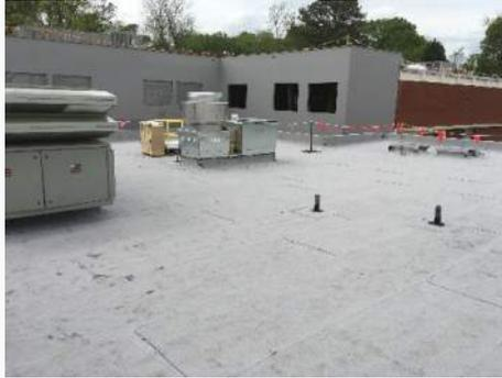
Installing Roofing Cap Sheet
